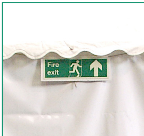
3K • Fire Exit Sign
