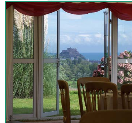
10D • Fire Exit Doors
